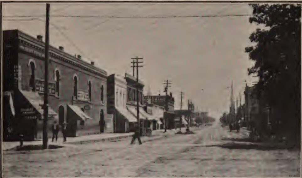
The business blocks are of brick, mostly two and three stories
